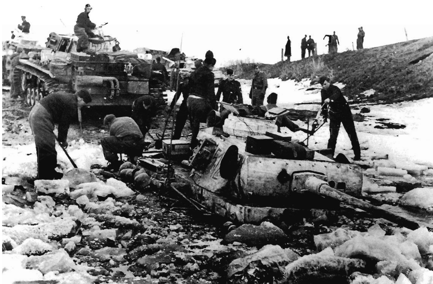
A Pz.Kpfw.III Ausf.M being retrieved by another Pz.Kpfw.III Ausf.M after it had broken through the ice while attempting to cross a river during the offensive to retake Kharkov. (BA)
