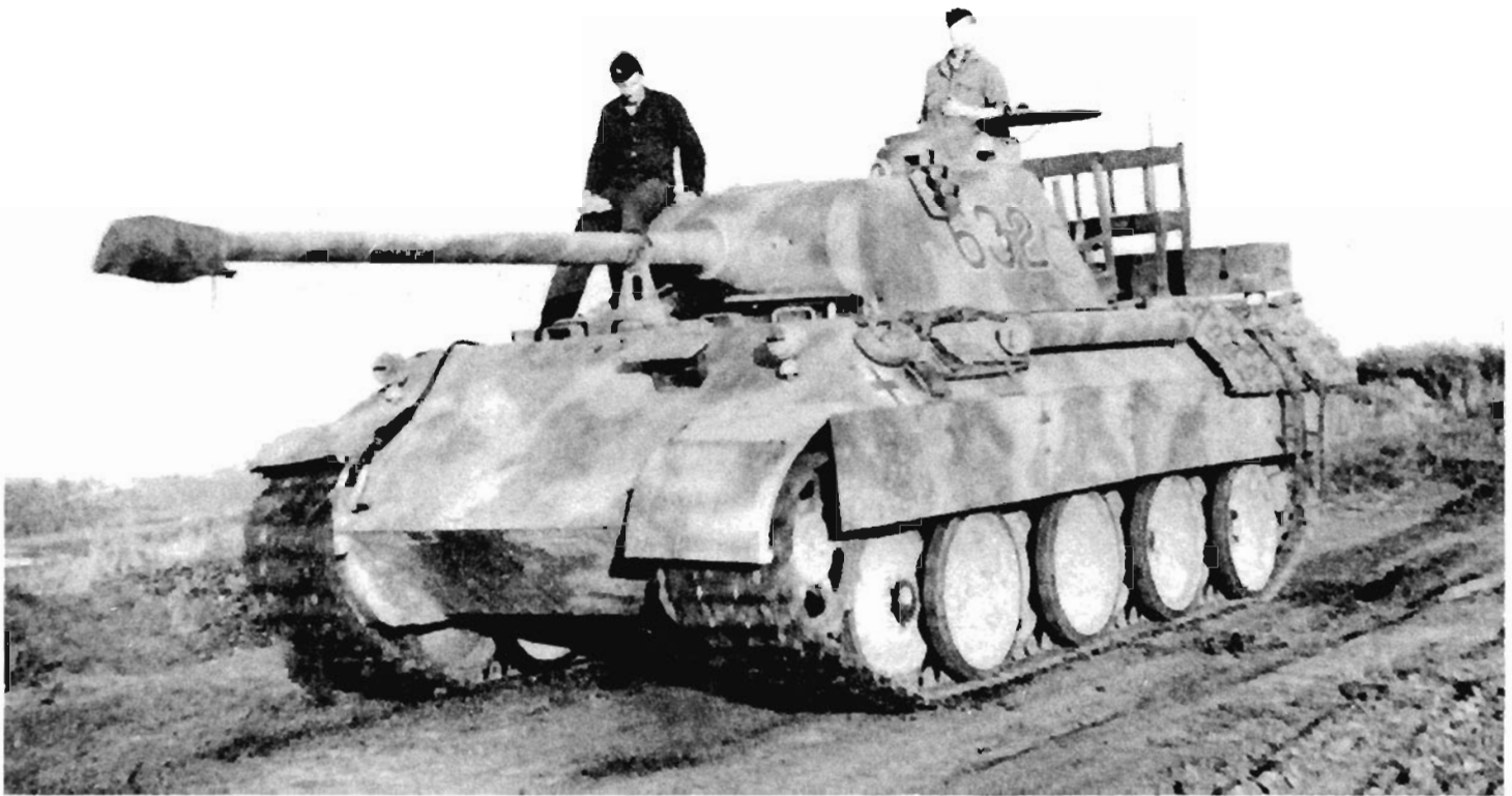
A Panther Ausf.D from the 2.Kompanie/Panzer-Abteilung 52 moving forward to an assembly area. While the launchers are still mounted on the turret side, there aren't any Nebelkerzen (smoke candles) in them. Use of this device had been discontinued following reports of crews being incapacitated when the Nebelkerzen were set off by hits from small-arms fire. (KHM)
